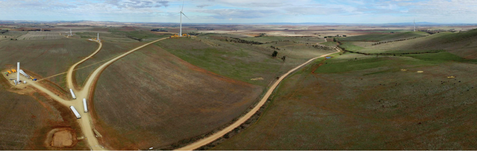
Figure 3: Hornsdale wind farm under construction.
